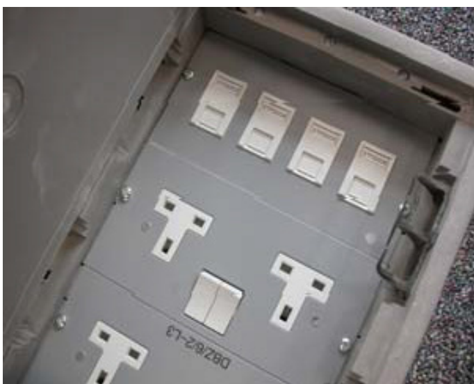
Floor box with four LJ6C modules
