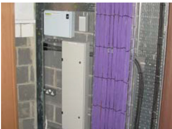
Finished riser on the first floor
